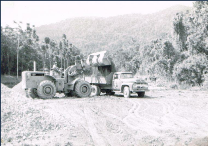
Image 17 © Brian Mundy Collection 2020 Jarrah Creek Camp 1967: this front-end loader is shown loading up the International Tipper with sand for the roadworks.
