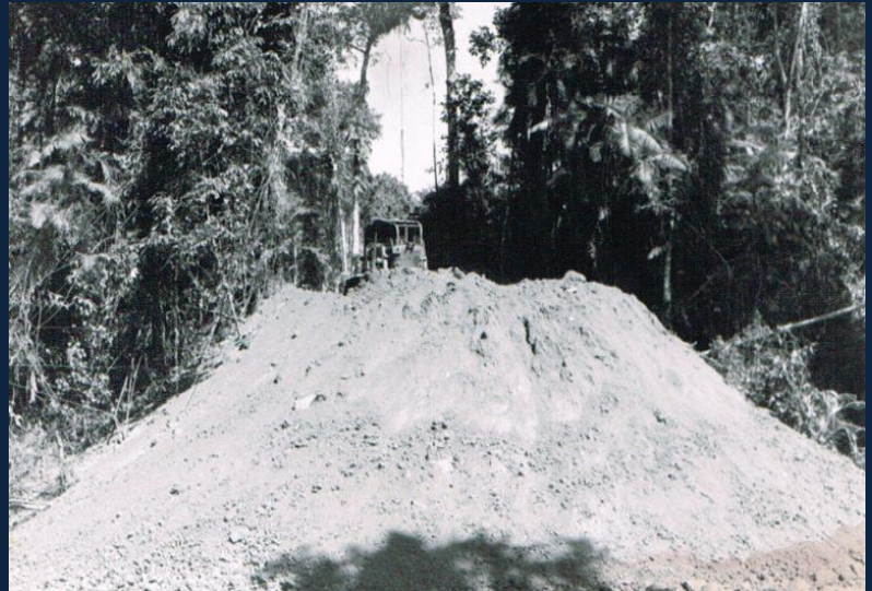
Image 13 © Brian Mundy Collection 2020 Jarraah Creek Camp 1967: the sandy soil was heaped up and used for finishing the road into the training area.
