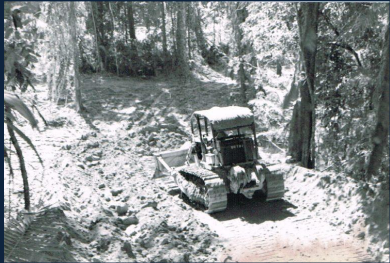
Image 10 © Brian Mundy Collection 2020 Jarraah Creek Camp 1967: a Caterpillar D4 or D7 is shown clearing the scrub to extend the training area
