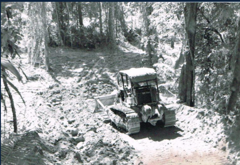
Image 11 © Brian Mundy Collection 2020 Jarraah Creek Camp 1967: a Caterpillar D4 or D7 is shown clearing the scrub to extend the training area
