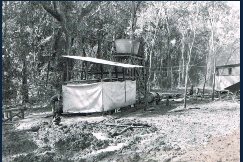
Image 7 © Brian Mundy Collection 2020 Jarraah Creek Camp 1967: the latrines and shower block built by the Troop. The overhead tanks supply water for the showers; these would be filled daily by the Squadron's water truck.
