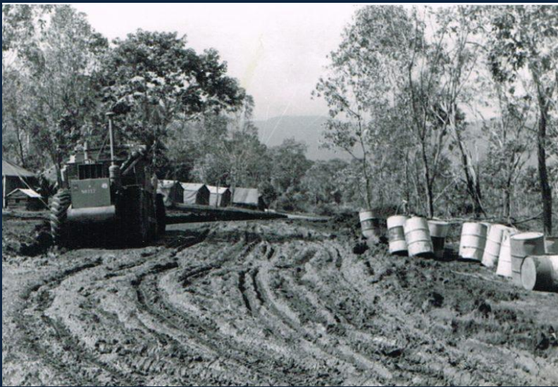
Image 9 © Brian Mundy Collection 2020 Jarraah Creek Camp 1967: the Euclid scraper is shown grading the road through the camp.
